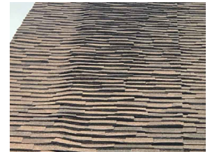
Pool Roof System (Exterior)
